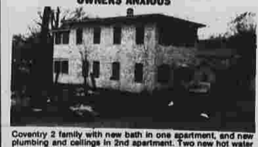
Coverly 2 family with new bath in one apartment, and new plumbing and ceiling in 2nd apartment. Two new hot water heaters. 2 bedrooms in each unit. Great income property! $89,900
